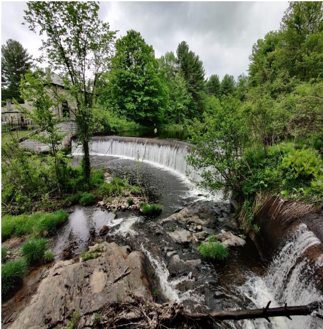
Quinepoxet Dam, W. Boylston, MA
